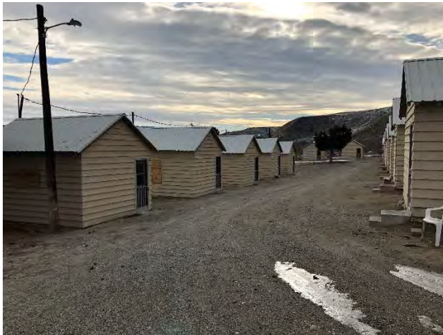
Figure 11: Farmworker Housing, Hwy 153 Near Pateros
